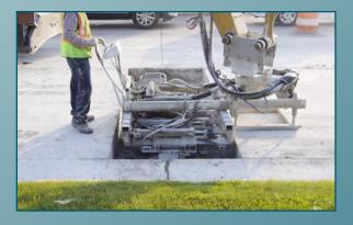
PCA drills also have a patented quick-release drill steel retainer that is easy to operate but doesn't open until you want it to. No more drill bits left in the hole because the retainer opened by itself!
